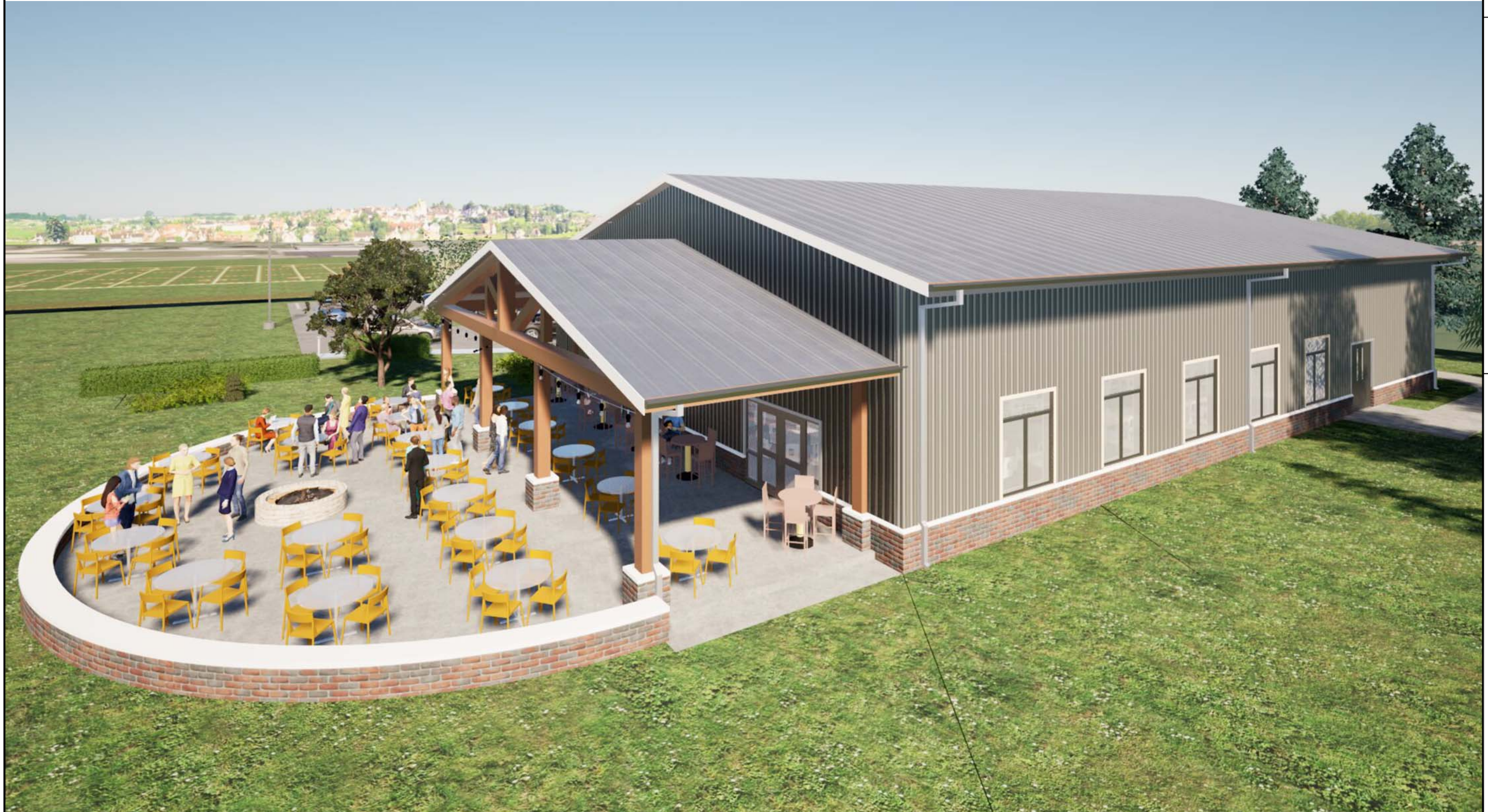
PRELIMINARY VIEW FROM SOUTHEAST
